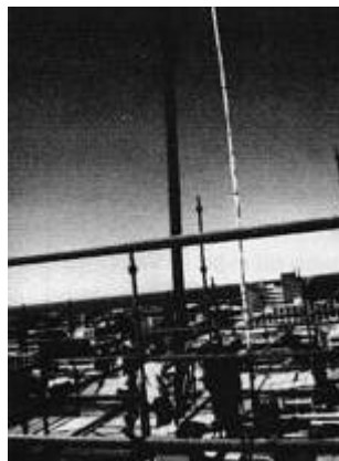
Figure 16: Vertical anchor installation by crane
