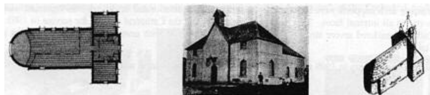
Figure 4: The remaining tower removed and bellcote added, circa 1868
